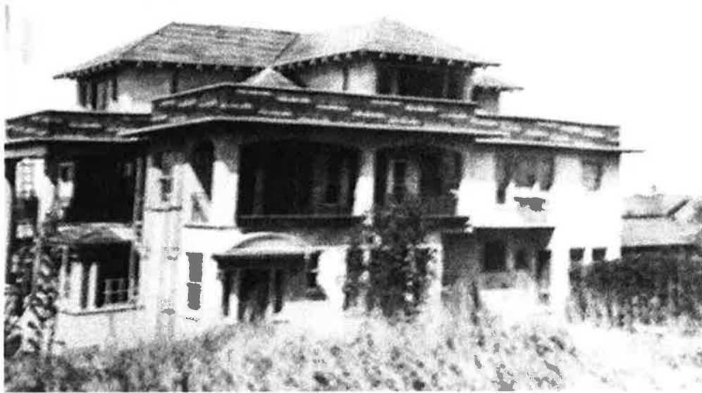
Axtell House after conversion to apartments showing extension of portico, additional wing, stucco treatment, modernized roof and windows created for Frances Axtell's conversion of her home into apartments. c. 1926. Photograph courtesy of William B. Hussey.
