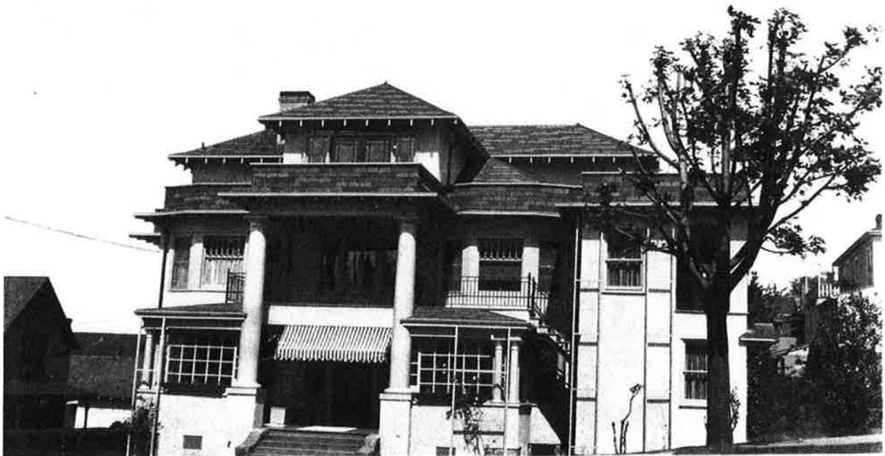
Axtell Apartments showing extension of portico, additional wing, stucco treatment, modernized roof and windows created for Frances Axtell's conversion of her home into apartments. c. 1927. Photograph courtesy of William B. Hussey.
